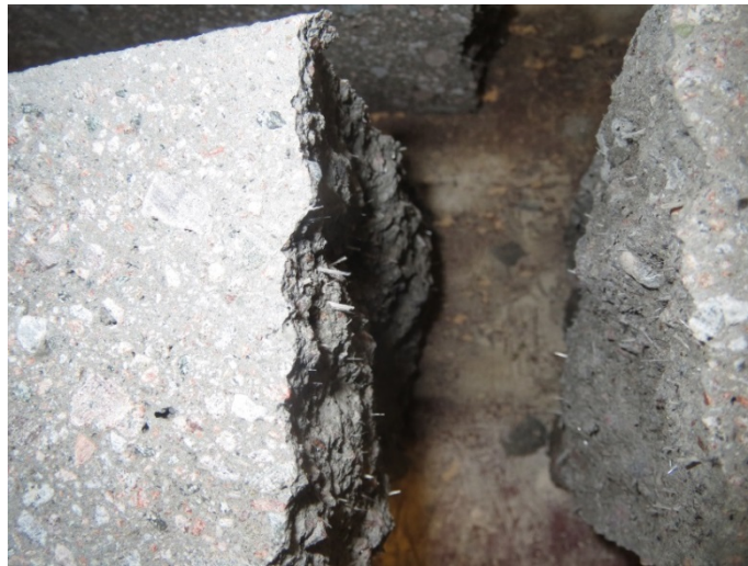
Figure 4.4. Glass fibre in failure surface of beam tested in bending.
