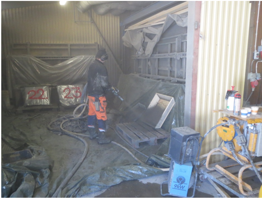
Figure 2.1. Operator spraying a test box with shotcrete, from which specimens for compression and flexural strength test were later cut out.
