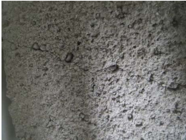
Figure 5.6. Crack formation in slab no 2 showing large aggregate impact pattern.
