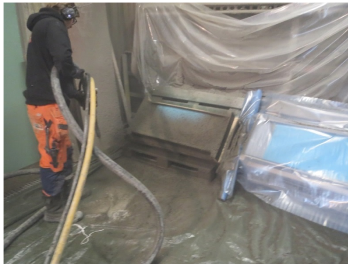
Figure 4.13. Spraying of test slabs.
