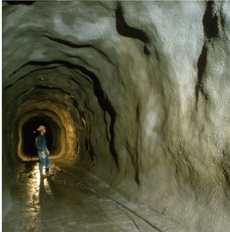
Figure 1.1. Tunnel lining of steel fibre reinforced shotcrete. Picture by courtesy of BESAB, Gothenburg, Sweden.
