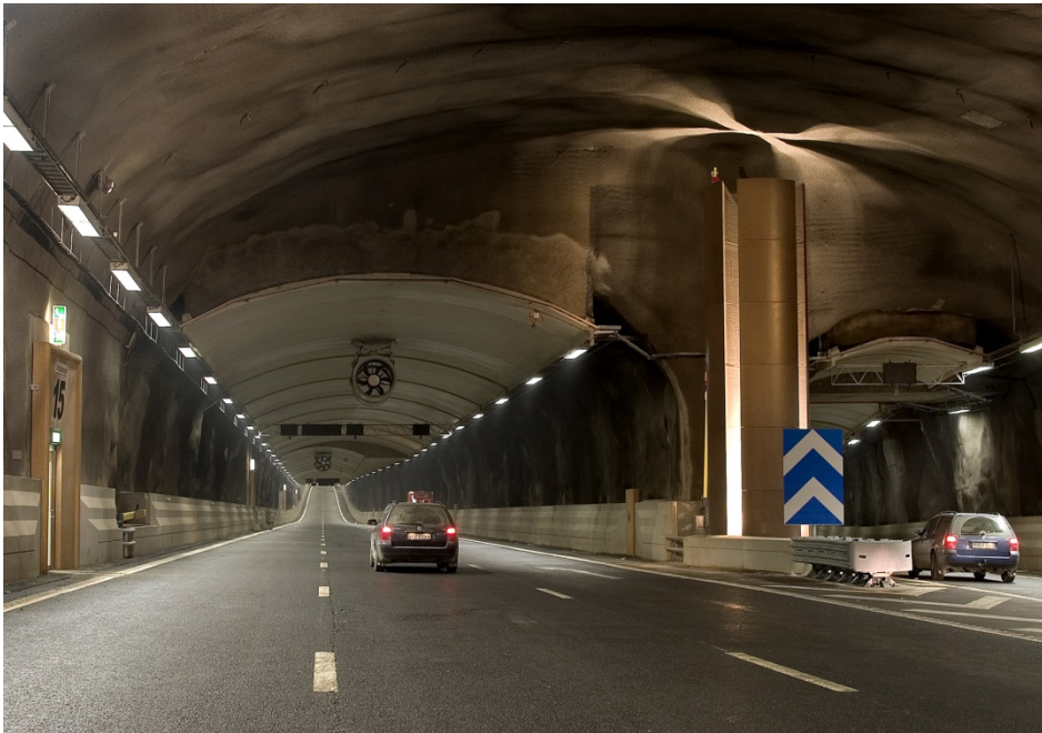
Figure 2.7. The Southern Link road tunnels, constructed with shotcreted drains. Photo provided by the Swedish Road Administration.
